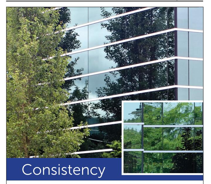
All glass that is subjected to the heat treating process will have some degree of distortion. Poor control of this process can increase distortion significantly (see inset).
